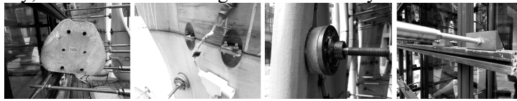
Figure 4. Mortise & Tenon (left); Metal plate (middle left); Ball joint (middle right); Rod and slider (right).
