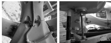
Figure 6. One joint condition (left); inflexible connection (right).
