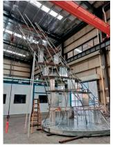
9 Offsite test assembly using CNC-cut recyclable metal sheet guides to accurately position and fix pipes with swivel shackles [Program Contractors Ltd. (PCL), 2021 ©].
