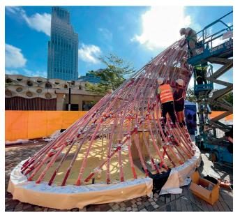
$\textbf{11} \ \ \textbf{Onsite reassembly using CNC-cut guides to position pipes [Laboratory for Explorative Architecture \& Design Ltd. (LEAD), 2021 ©]}.$
