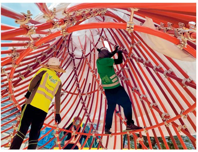
12 Onsite reassembly using CNC-cut guides to position pipes [Laboratory for Explorative Architecture & Design Ltd. (LEAD), 2021 ©].
